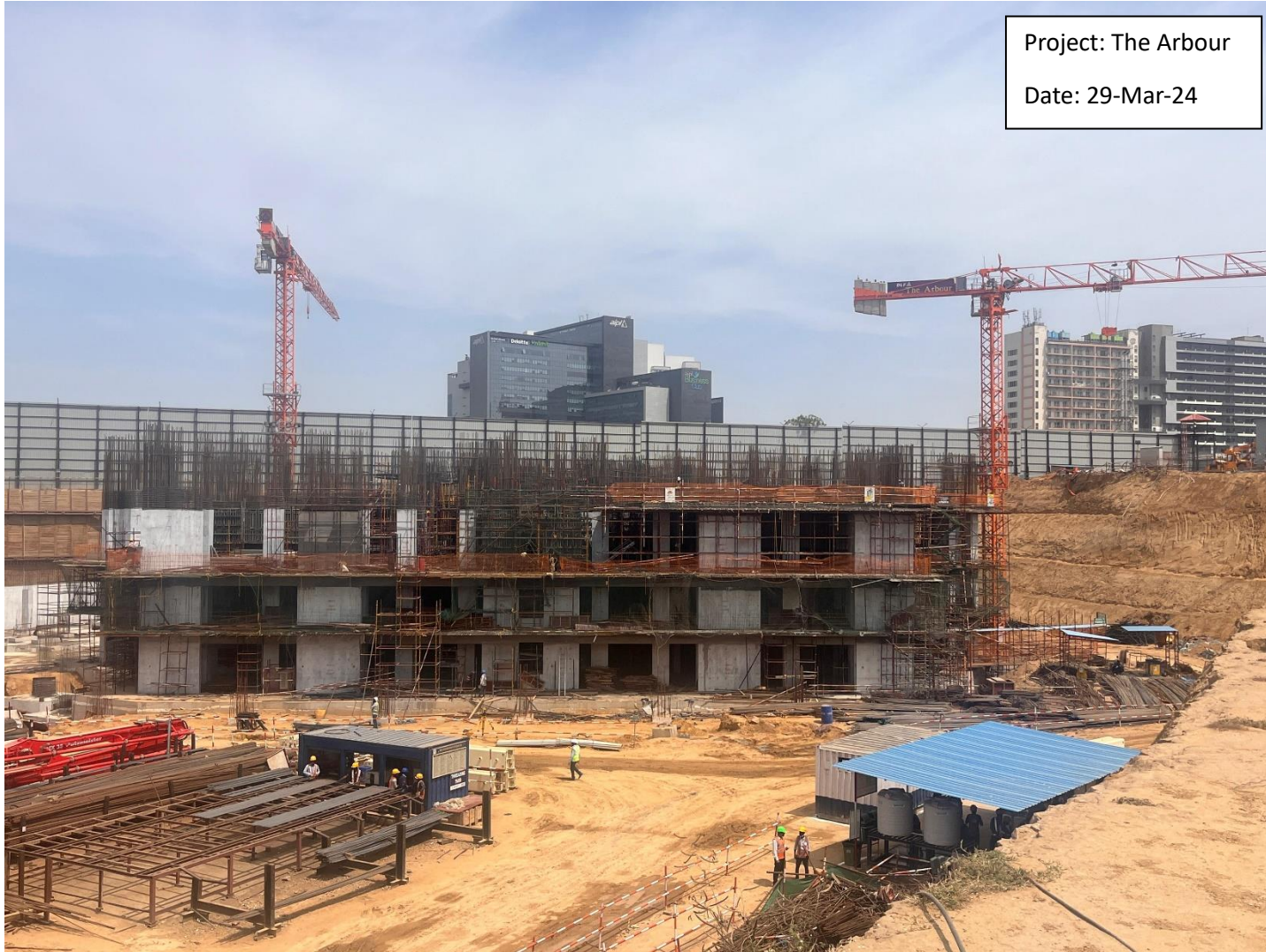
Tower C – B1 Slab completed, GF WIP
