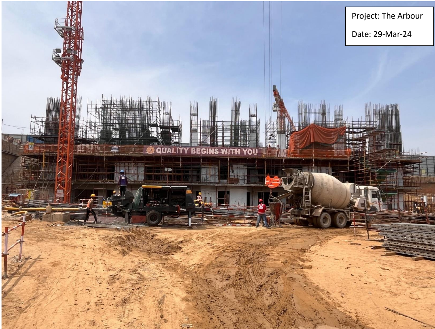
Tower A – B2 Floor Slab completed, B1 level WIP
