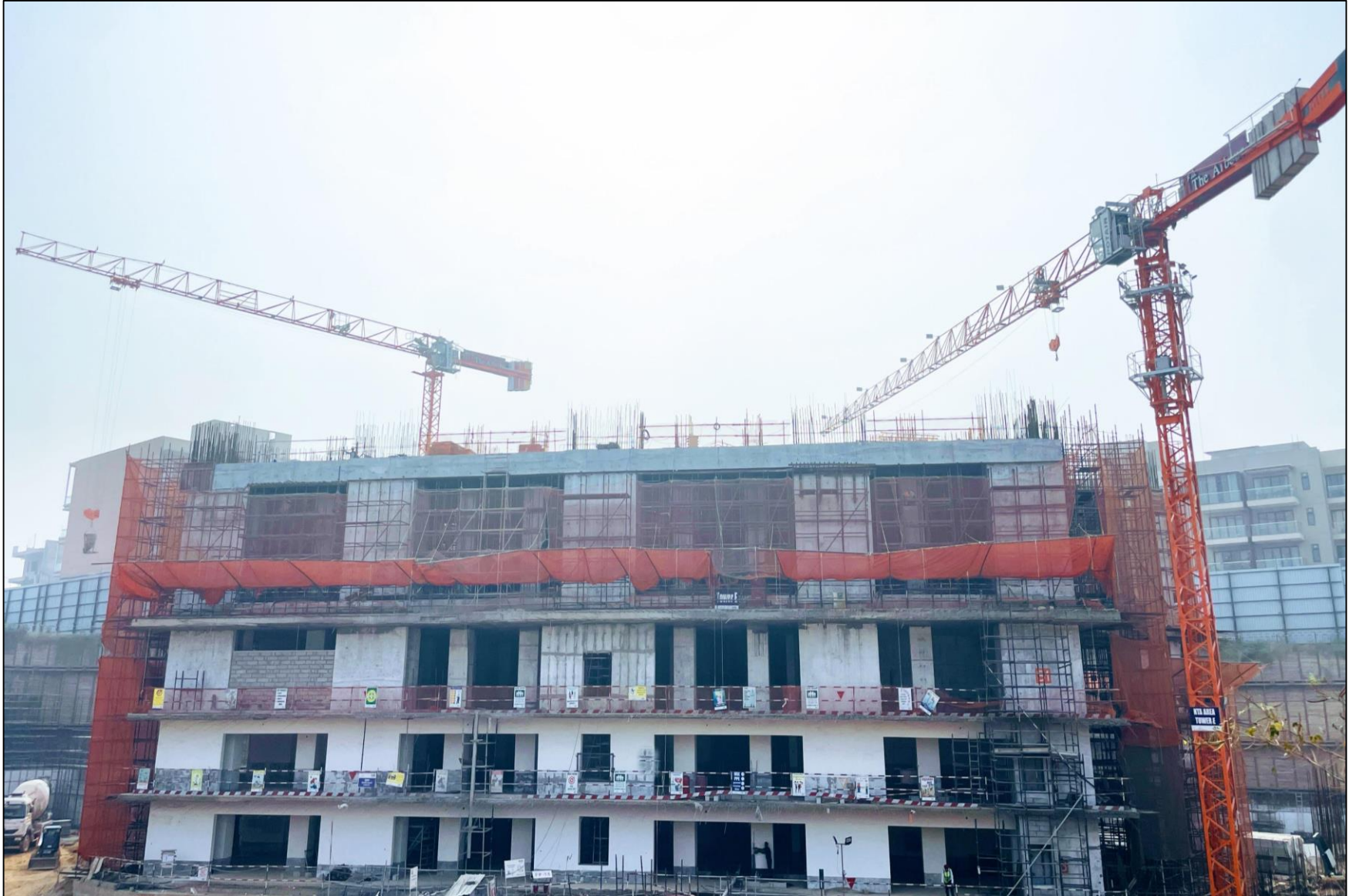
Tower E – 1F slab WIP
