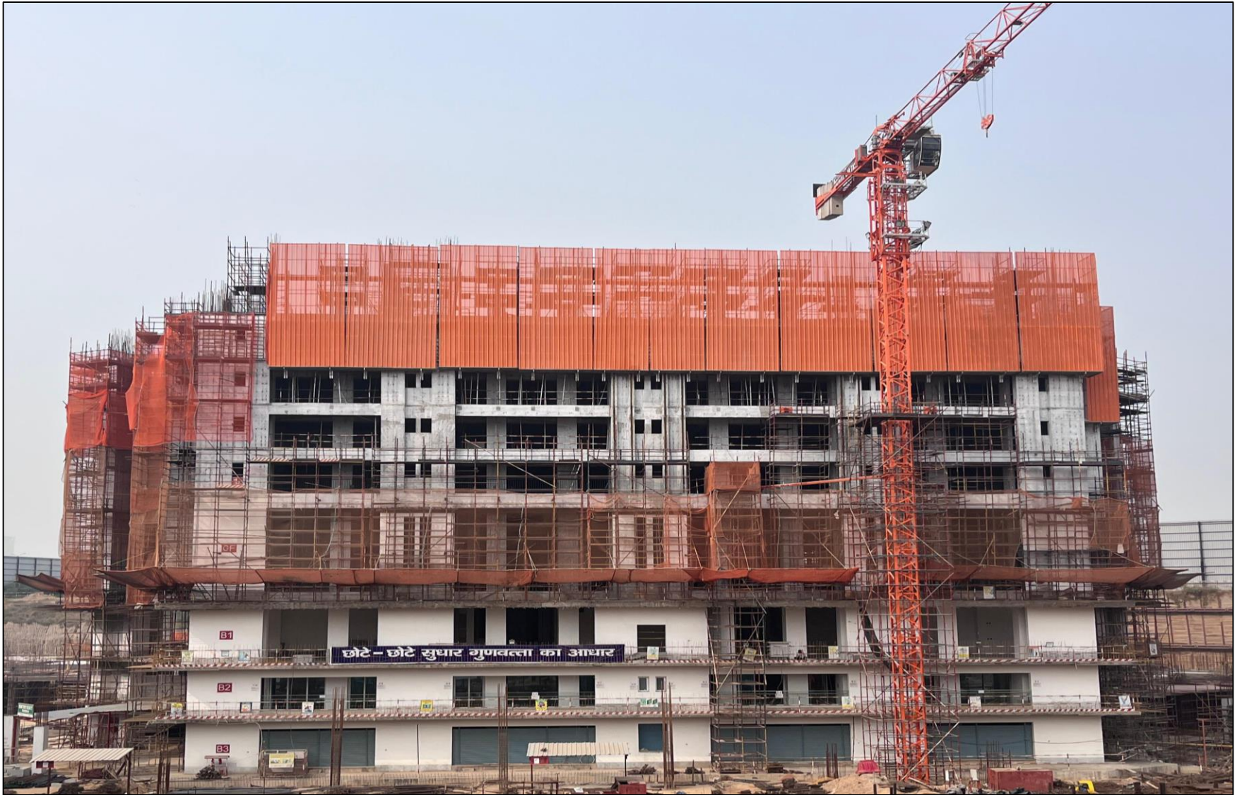
Tower B – 5F & 6F Verticals WIP
