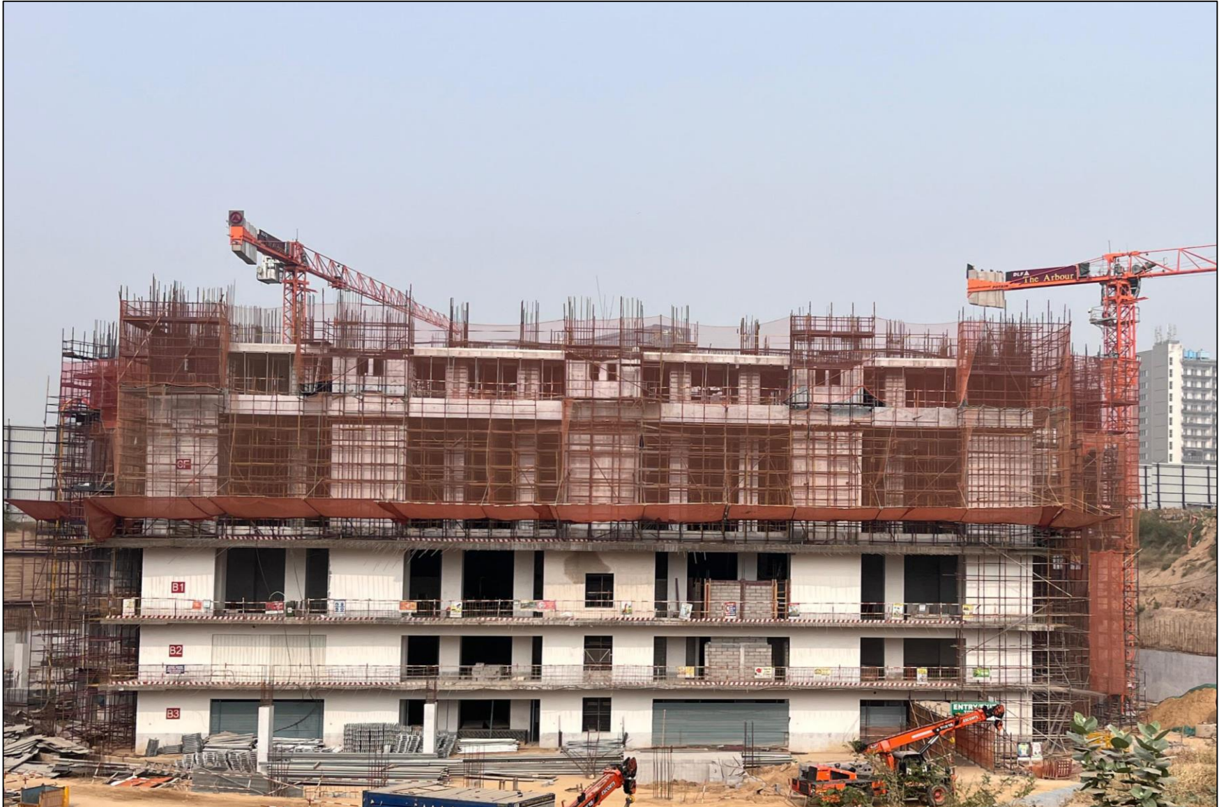
Tower C – 2F Verticals & Formwork WIP
