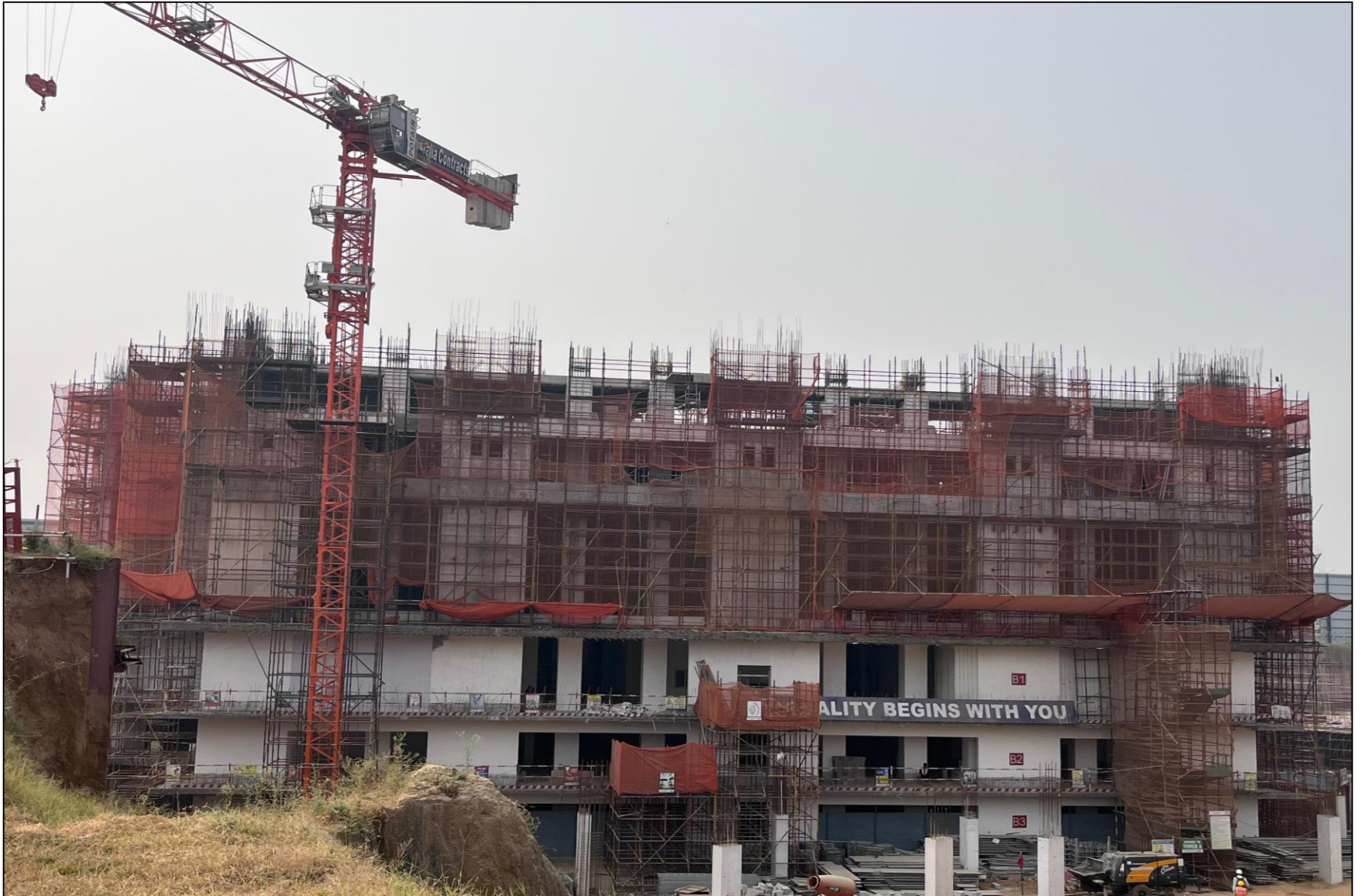
Tower A – 2F slab WIP
