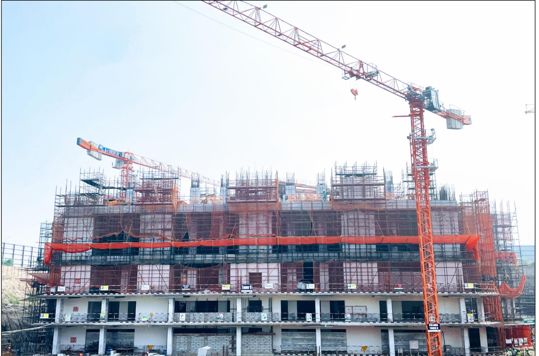
Tower D – 2F slab WIP
