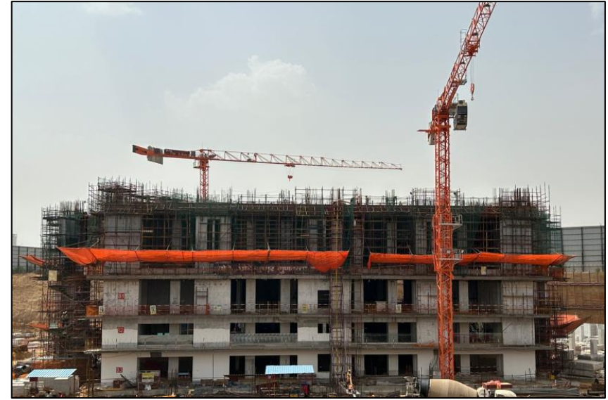
Tower B – 1F Slab WIP
