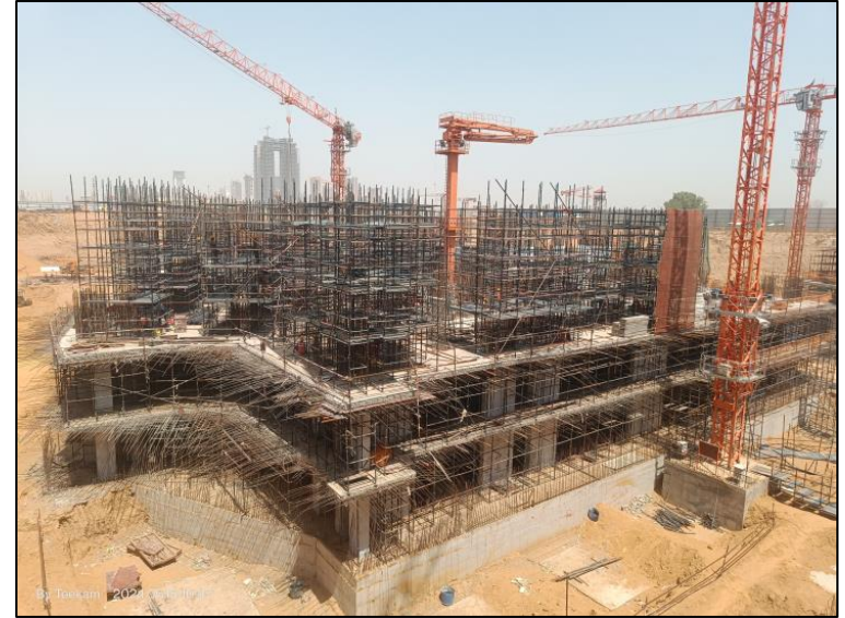
Tower E – GF Slab WIP
