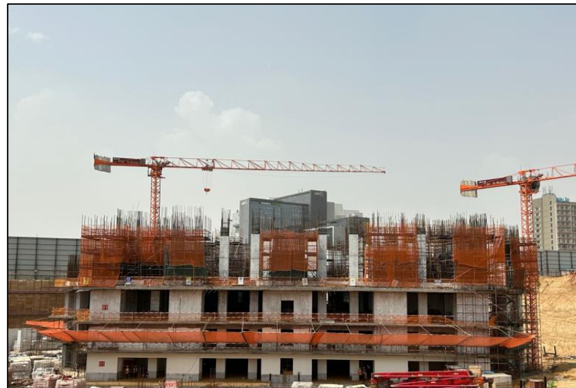
Tower C – 1F Slab WIP
