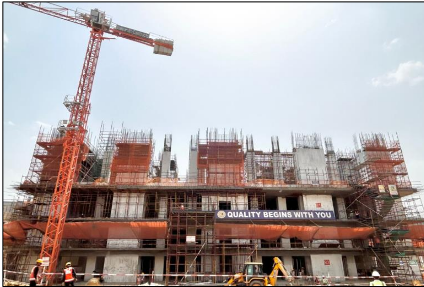
Tower A – 1F Slab WIP
