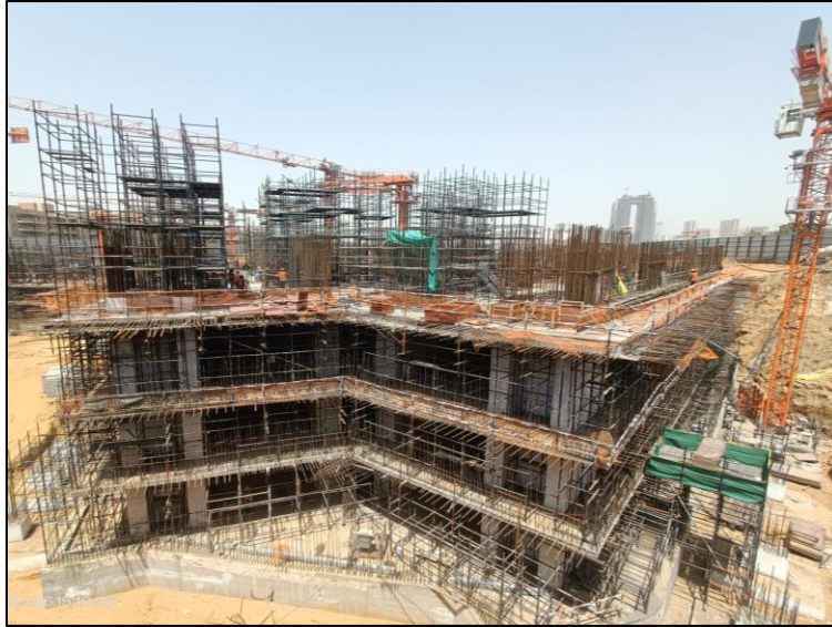
Tower D – 1F Slab WIP
