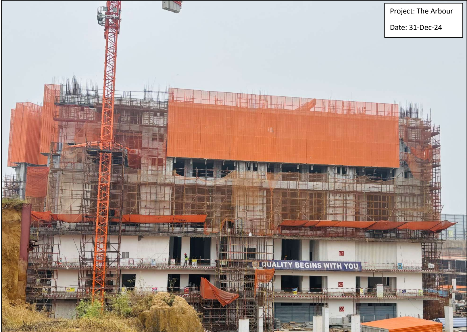
Tower A – 3F Slab WIP
