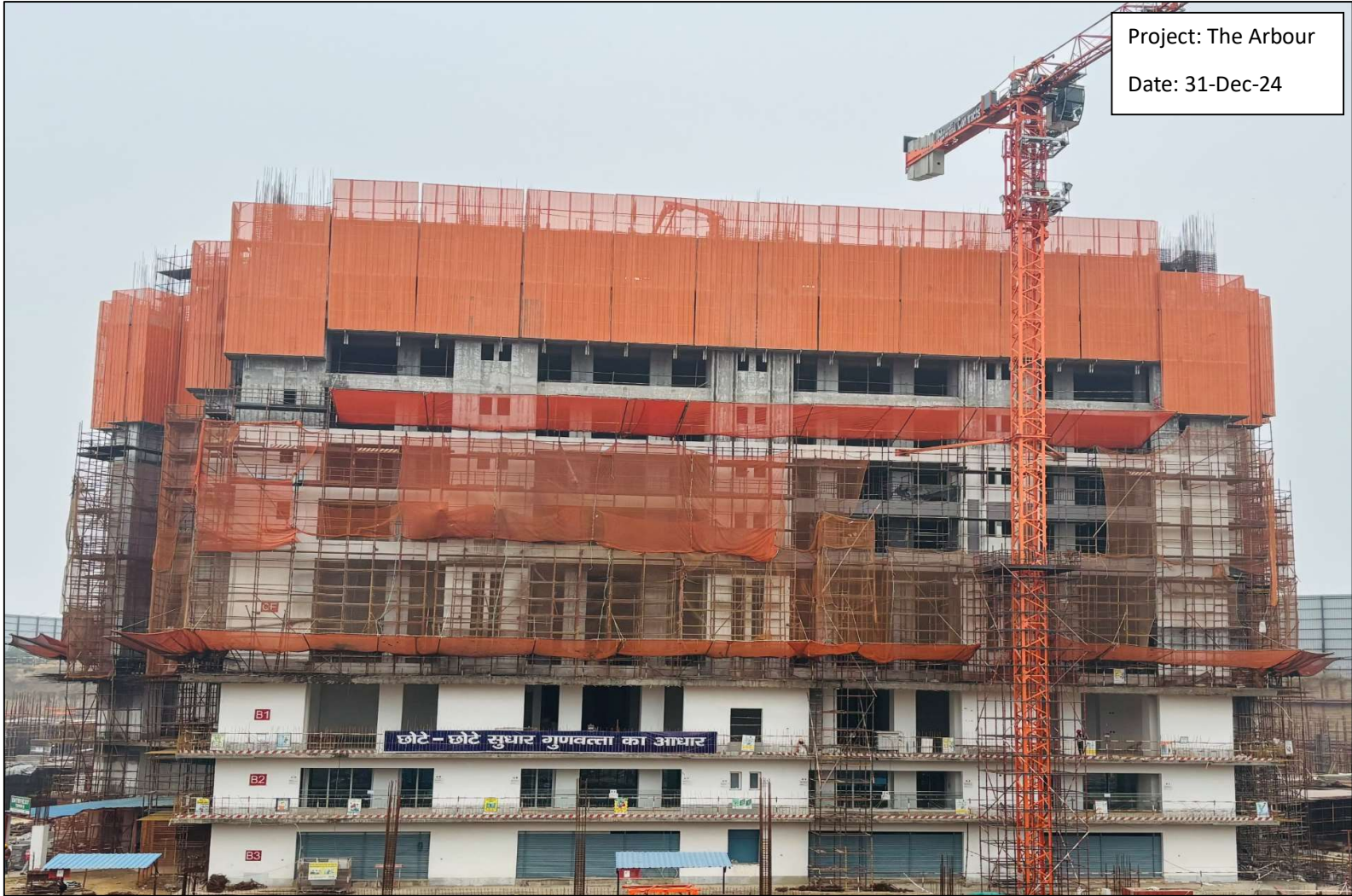
Tower B – 6F Slab WIP
