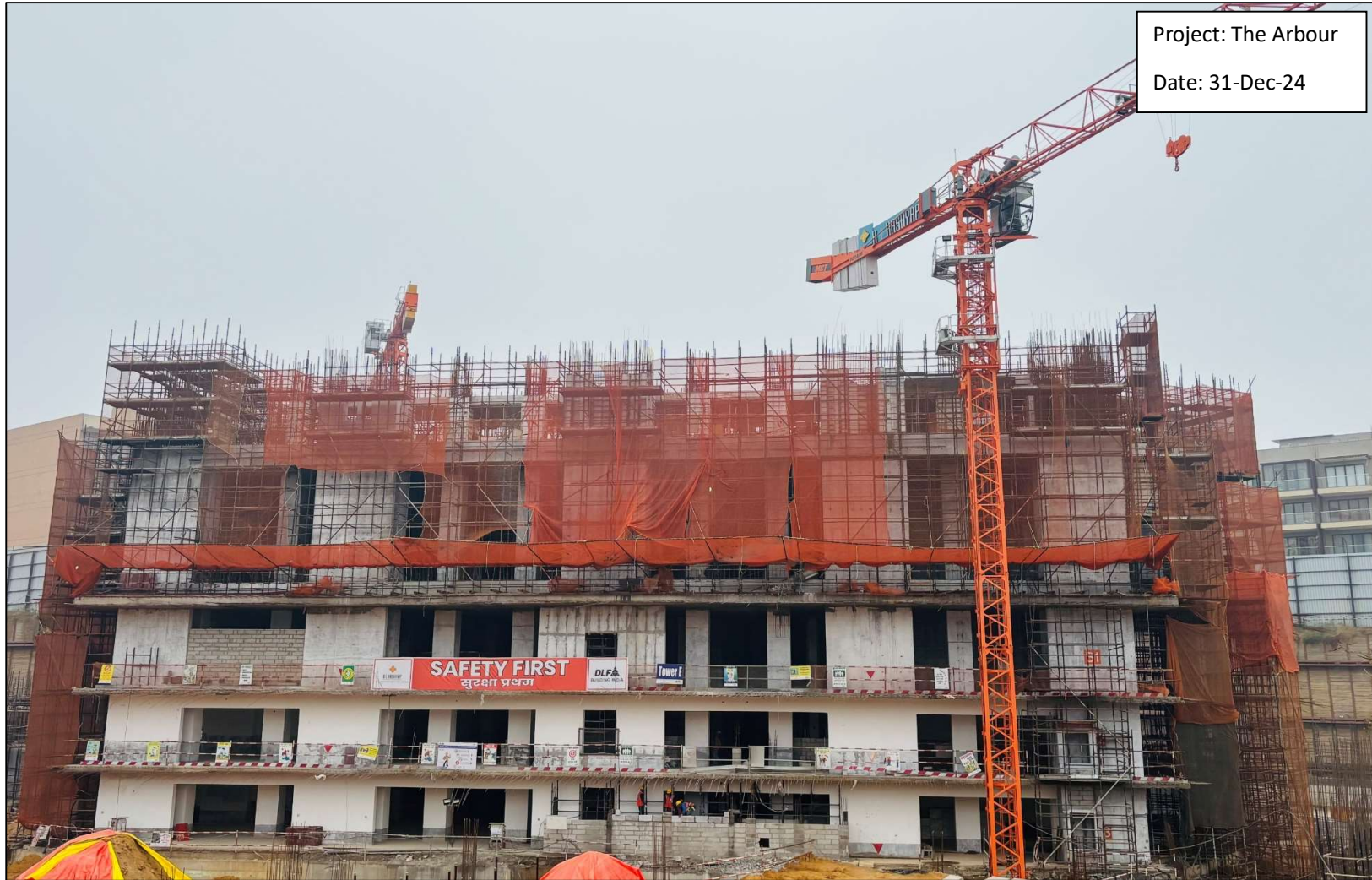
Tower E – 2F Slab WIP
