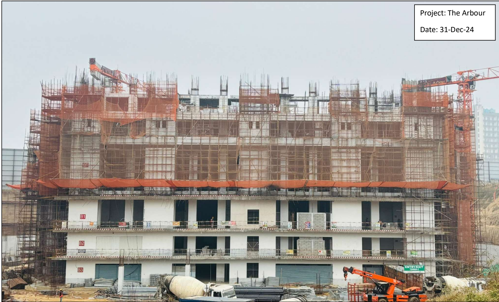
Tower C – 2F Slab WIP
